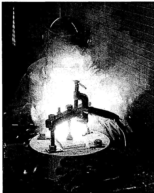
Figure 7.8: Outdoor Welding of Galvanized Steel
